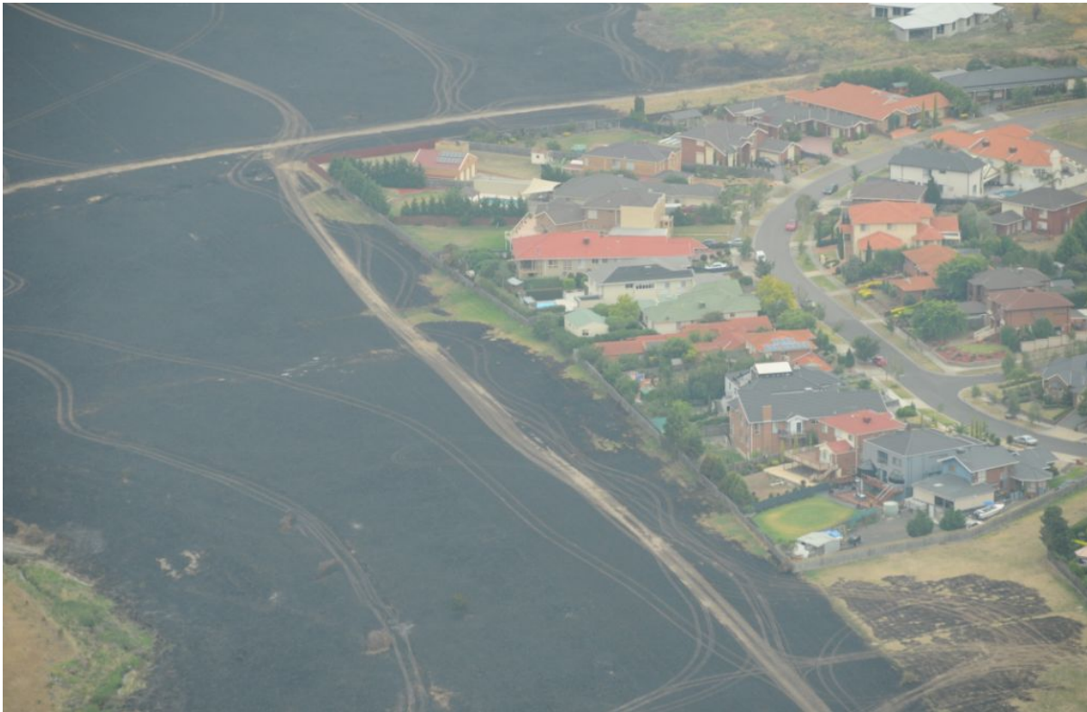
Figure 3. About the middle of the fire, showing the benefits of an internal track and slashing works between the track and boundary fences.
